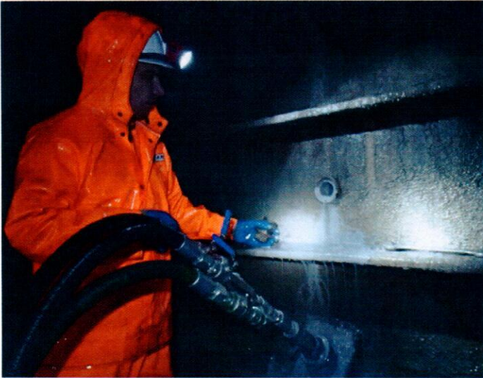
Pic. left: Shaft sinker while monitoring of the grouting process
