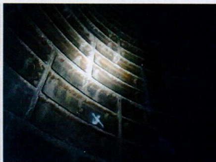
Leakage of grouting material between tubbings
