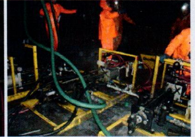
Pic. above left: Injection mounting for the sealing material "NOH2O"
