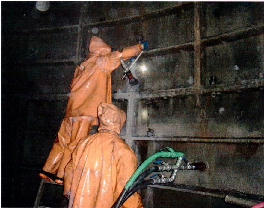
Pic. left: Shaft sinkers while grouting work inside the foreshaft
