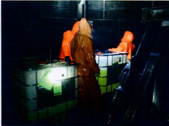
Chemical grouting material ready for the removal
